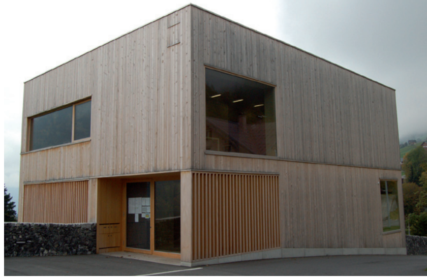
The municipal hall of St. Gerold in Großes Walsertal BR was constructed to passive-house standards. © BR Management
